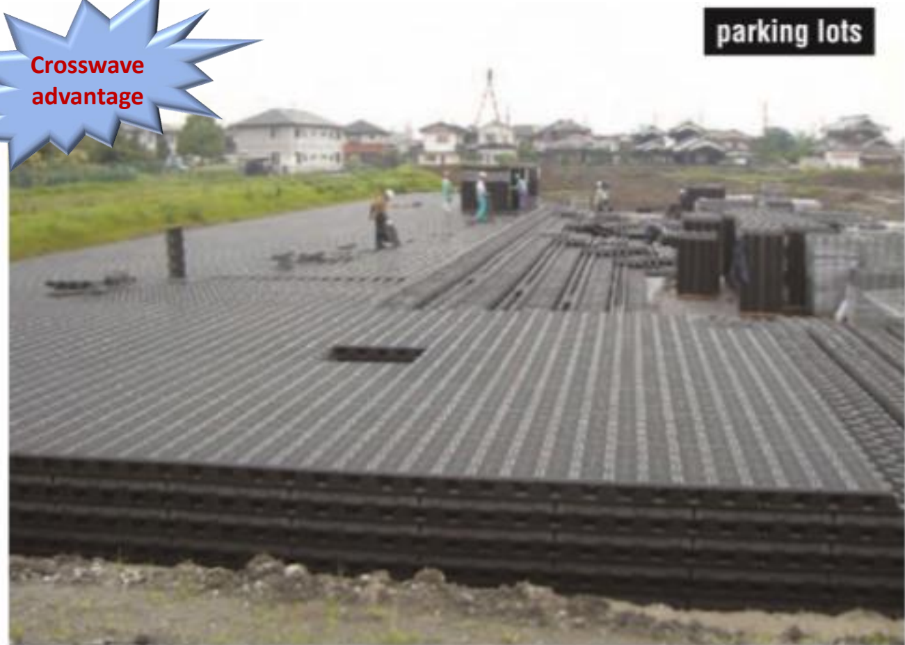
Rainwater regulating reservoir construction in Ehime prefecture, under the parking lot, at shopping centre (Storage capacity:6,600m 3 )
