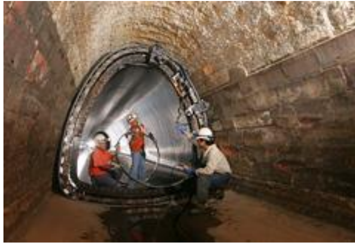
Sewer Pipe Rehabilitation
